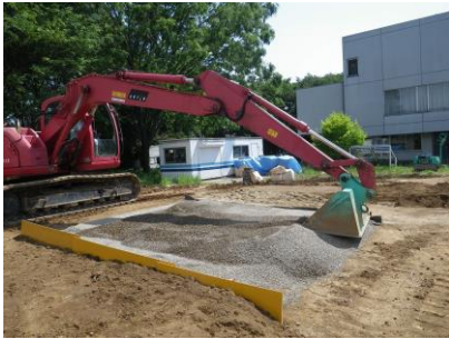
a. Gravel layer compacted by the plate-type bucket.
