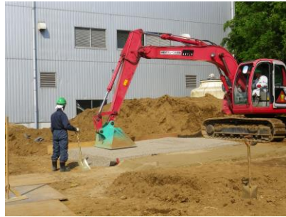
b. Sand layer compacted by the plate-type bucket.
