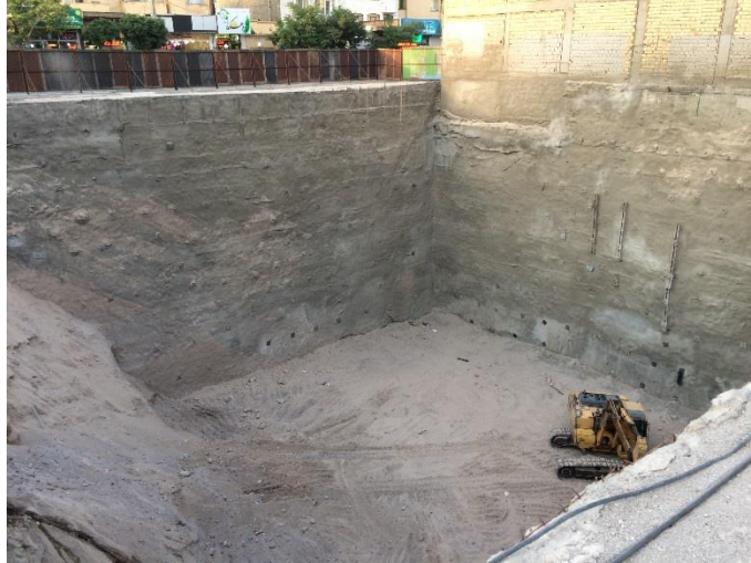
Fig. 4: The view of soil nail wall.
