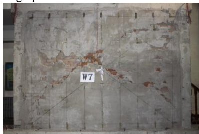
g) Damage photo of wall W7
