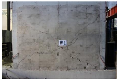
a) Damage photo of wall W1
