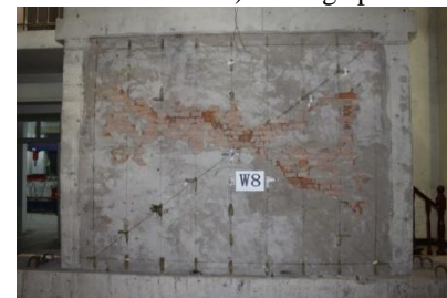
h) Damage photo of wall W8
