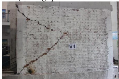
d) Damage photo of wall W4
