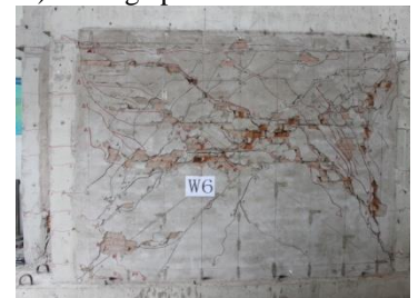
f) Damage photo of wall W6
