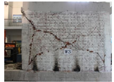
c) Damage photo of wall W3
