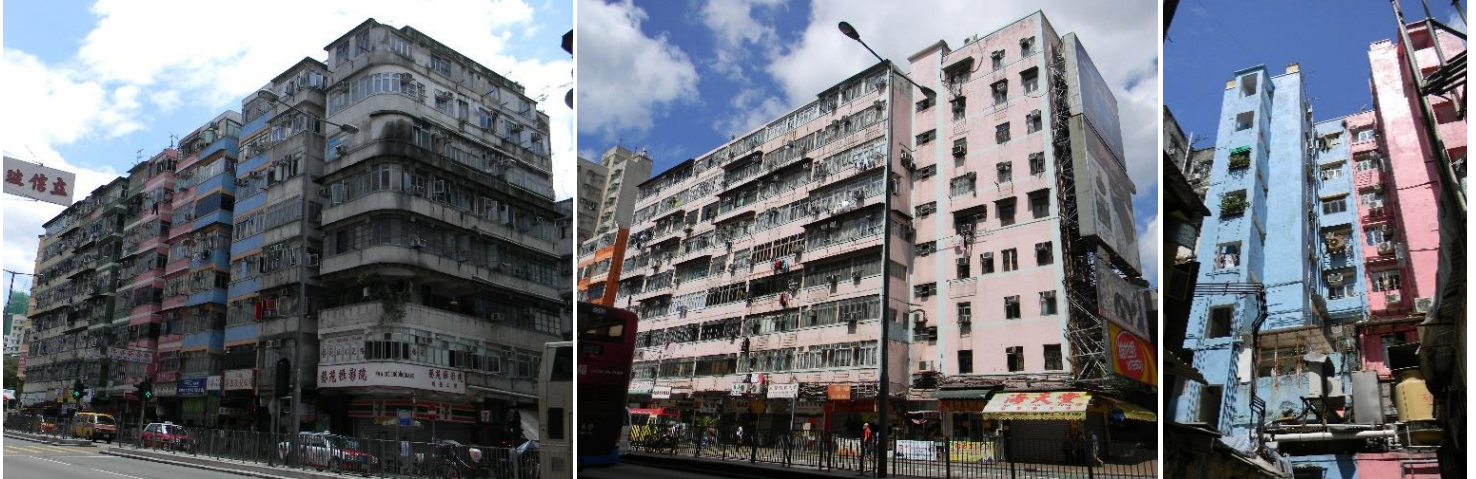
Fig. 2: No separation between the buildings in old districts (e.g. in Kowloon).
