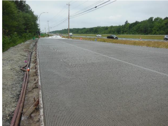
Fig. 7: PCCP view south to approach ramp showing tined surface.
