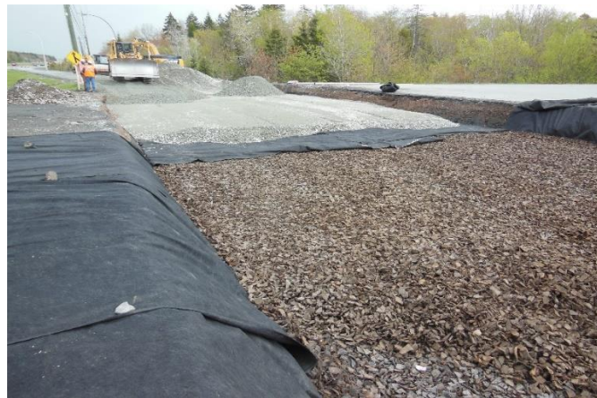
Fig. 5: Compacted TDA with type 2 subbase material placement occurring.
