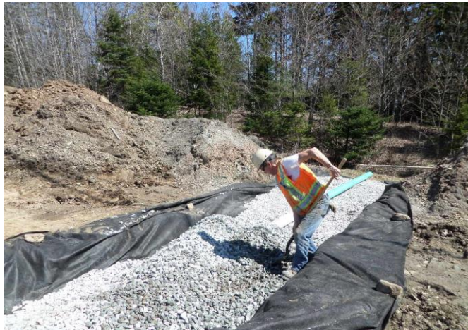
Fig. 4: Clear stone and perforated pipe drain installation.
