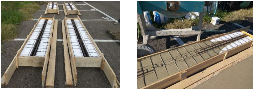
Fig. 4: Specimen formworks and casting.
