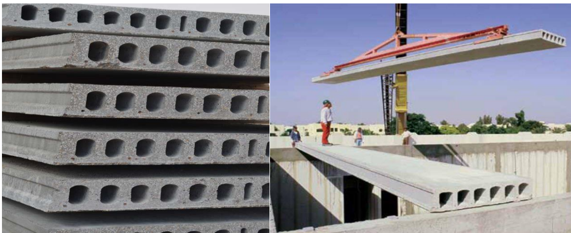
Fig. 2: Prefabricated hollow slab.
