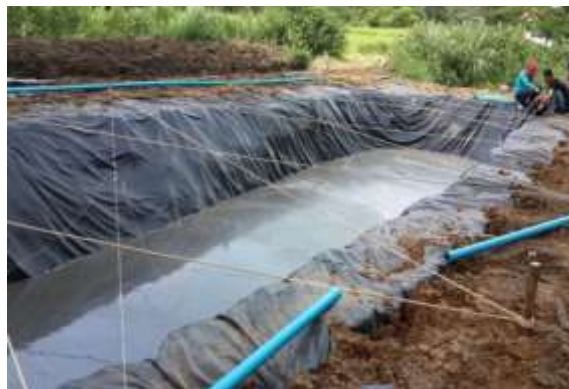
Fig. 2: The construction of wastewater lagoon digester.
