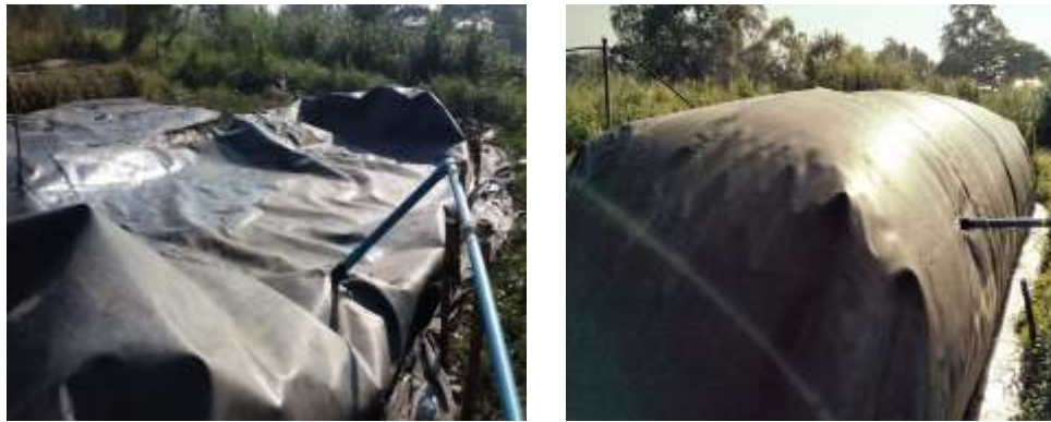
Fig. 3: Modified Cover Lagoon Digester (MCLD) before (left) and after (right) gas production.
