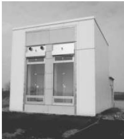
Fig. 2. Full-scale façade test facility (Cube) in Aalborg University.
