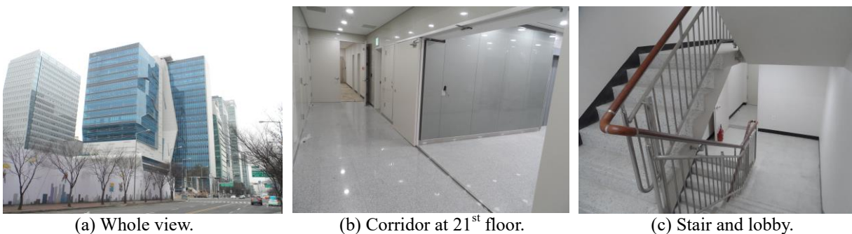
Fig. 1: Photograph of building structure.
