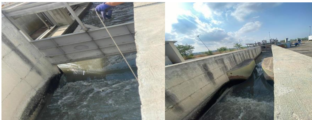
Figure 1. Pre - treatment sampling station
