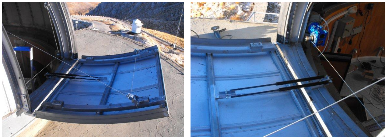
Fig. 5. The new design of the roof-shutter.
