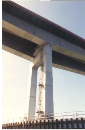
Fig. 1: Stiffened steel box bents of Hayward San Mateo Bridge in California (photo by Abolhassan Astaneh-Asl)
