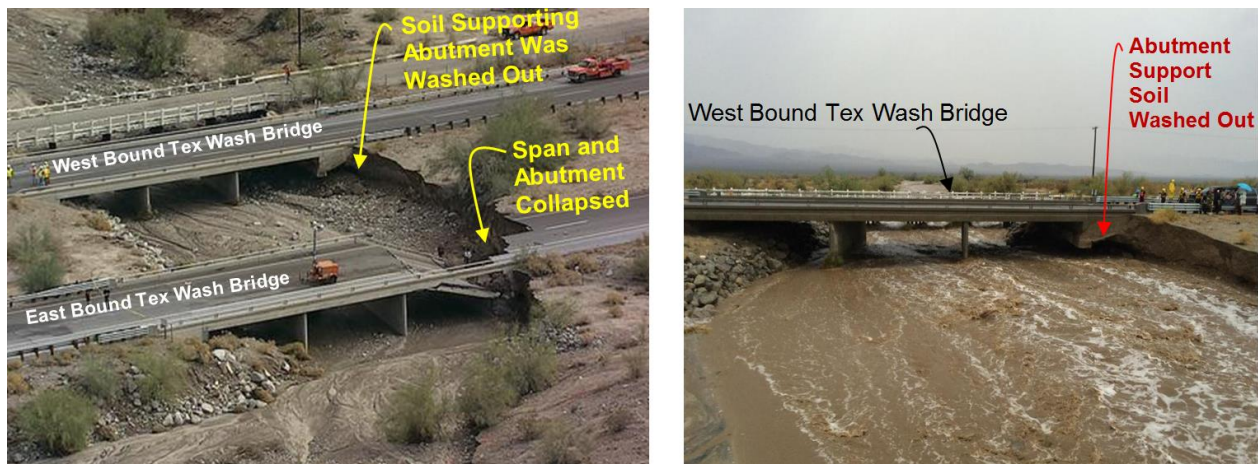
Fig. 4: Eastbound Tex Wash Bridge after Collapse.
