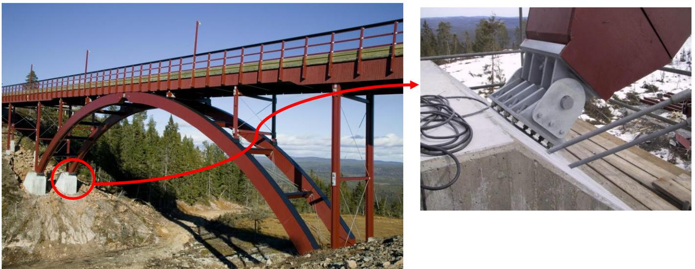
Fig. 29: Arch bridge of timber in Sweden. The total length of the bridge is 130 m, the span of the arch being 50 m. To the left a detail of the hinge at one of the springing points of the arch.
