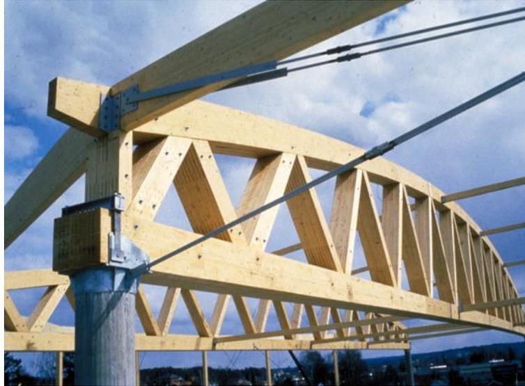
Fig. 17: Main truss of the Hamar olympic amphitheatre, Norway. The span is 71 m. The truss nodes consists of slotted-in plates and dowels (Photo: Moelven Limtre A/S).
