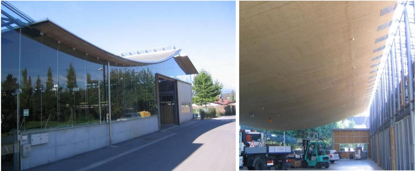
Fig. 31: Cable-shaped cross-laminated LVL roof in Switzerland. To the right, are visible the anchorages of the roof timber structure to the supporting steel structure by means of a number of nailed plate connections.
