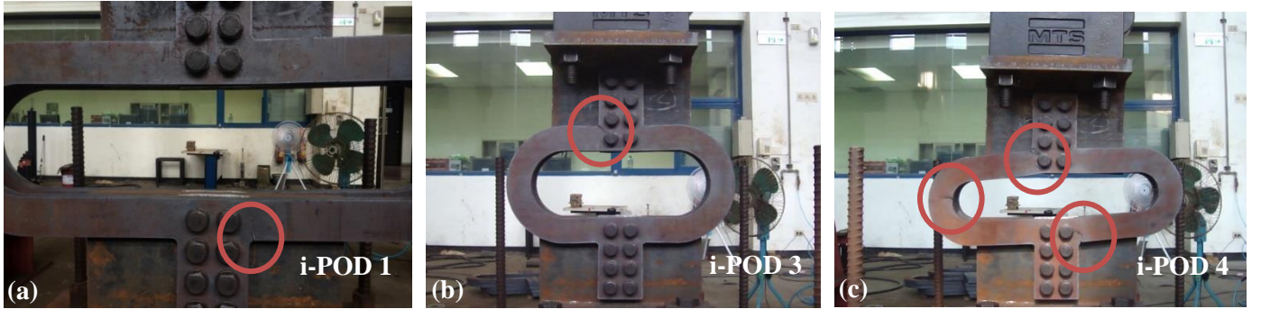
Fig. 6: Cracking locations of i-PODs at the ultimate states [13].
