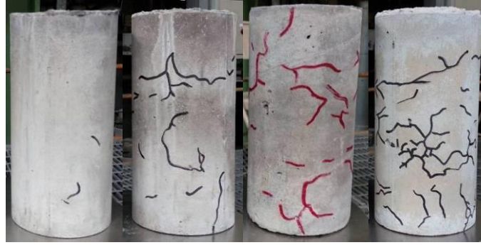
(a) 200 °C (b) 400 °C (c) 600 °C (d) 800 °C Fig. 10: Surface cracks of SCCPPF specimens using water cooling.
