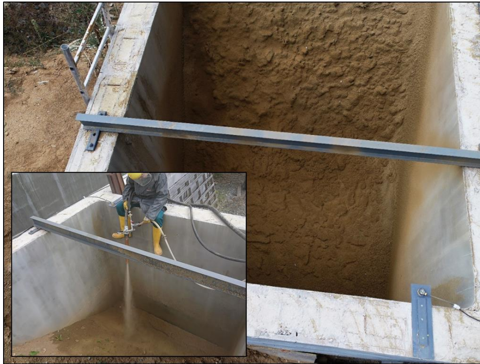
Fig. 5: Upstream face of the experimental dam with a bentonite layer applied and the application of bentonite (inside).
