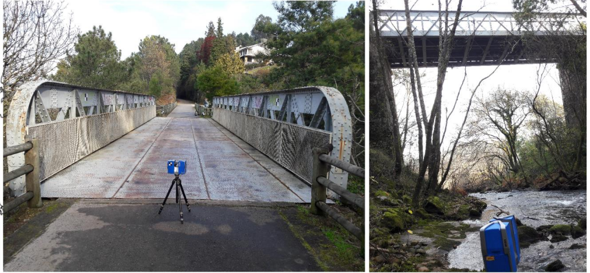
Fig. 2: Location and photographs of Lapela Bridge.
