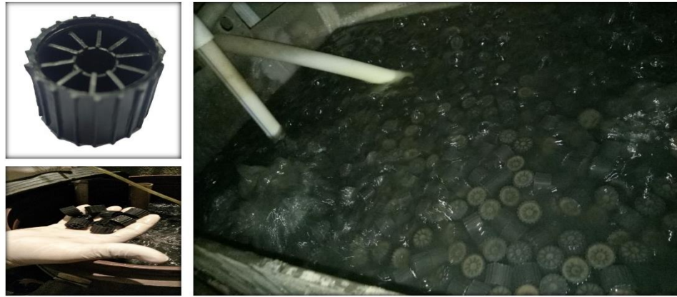
Fig. 2: Media used in the system with 50 % fill percentage in the tank.
