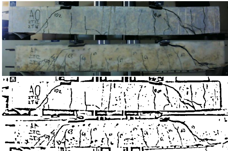
Figure 8: Real vs. Processed images of beams A0 and A1 to show the crack pattern and failure mode
