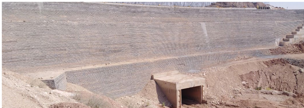
Fig 3: Reinforced embankment at the end of construction (Downstream View).
