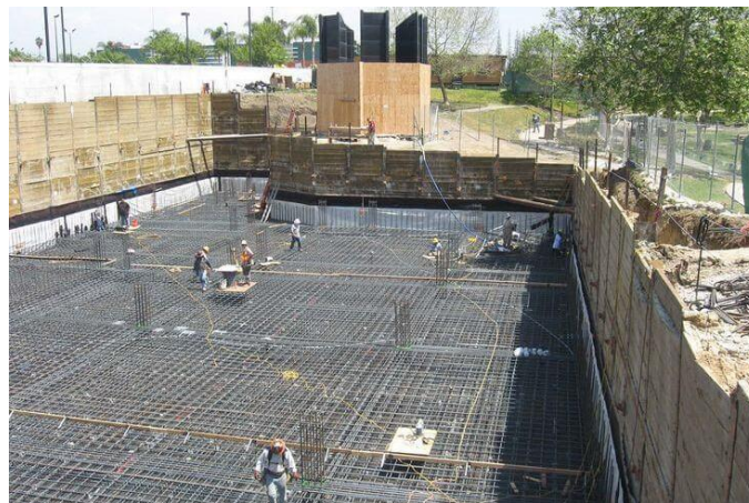
Fig. 1: Typical raft foundation under construction [1].
