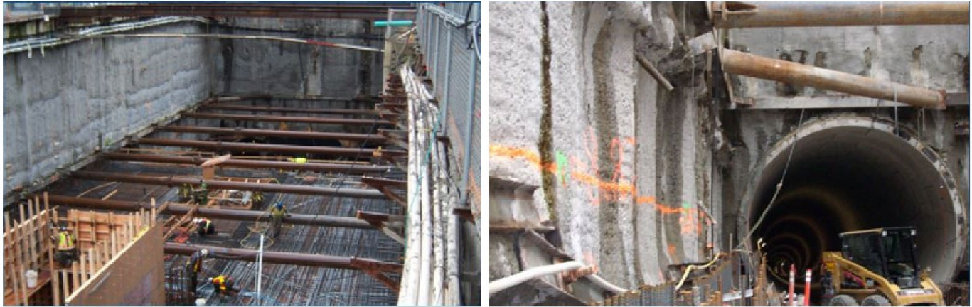
Fig. 4: Construction works of The Canada Line: Yaletown – Roundhouse [9].
