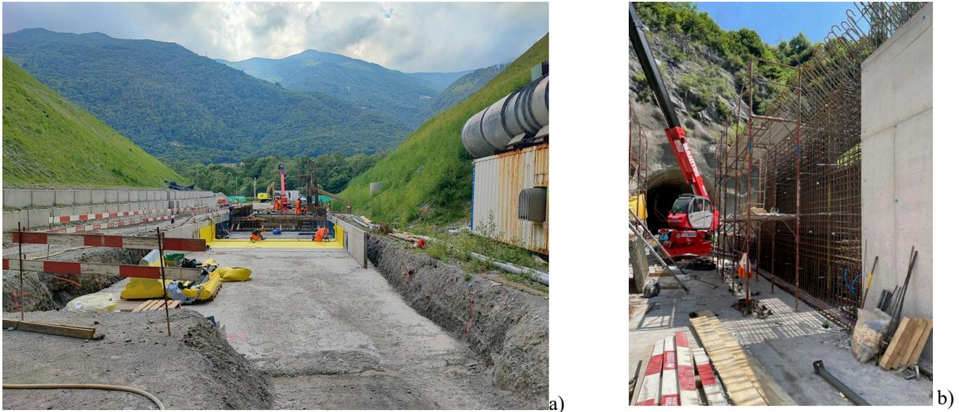
Fig 7: a) Steel reinforced slab construction; b) view of the steel reinforcement placement into the wall of the artificial gallery.
