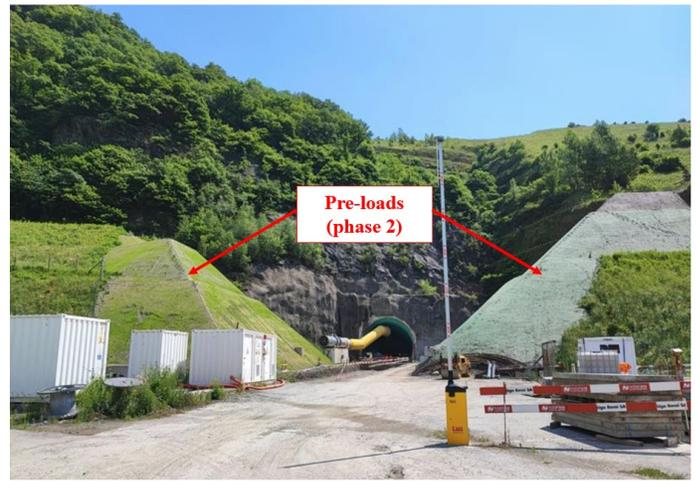
Fig. 5: a) Evolution of settlements over time the time by AS01-AS10 measurements; b) Lateral pre-loads, phase 2.
