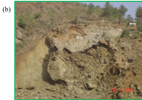
Fig. 3:a,b. View of slide in the u/s of powerhouse cut slope between RD -7m and +9m starting from El \pm 1440\text{M} to El \pm 1368\text{M}
