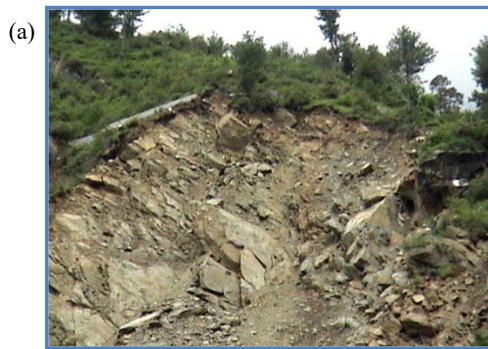
Fig. 3:a,b. View of slide in the u/s of powerhouse cut slope between RD -7m and +9m starting from El \pm 1440\text{M} to El \pm 1368\text{M}
