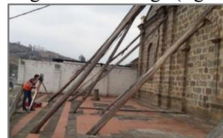
Fig. 2 Altimetric survey of rear wall.
