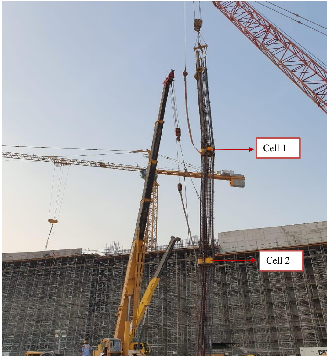
Fig.1: Cage installation of two –tier BDSLT
