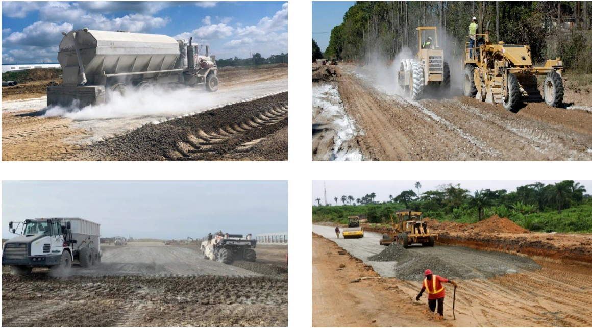
Fig.2 : Earth material stabilization and construction process in the field.
