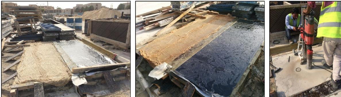
Fig. 5 Preparation of the blanket, curing process, and core drilling.
