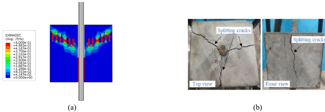
Fig. 3: Cracking pattern (a) FE model (b) Experimental sample [32]
