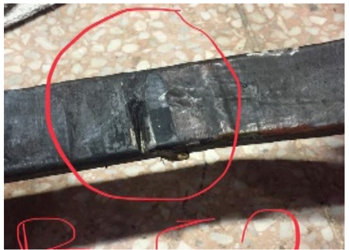
Fig. 6: Damage on Bar due to Lamination Piece
