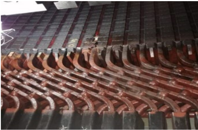
Fig. 1: Visual Inspection - Rotor Poles removed
