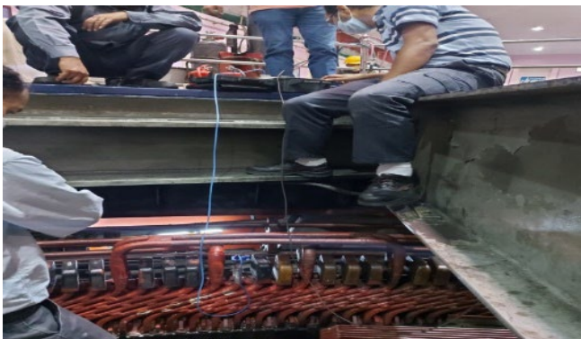
Fig. 3: Testing of Stator Sections
