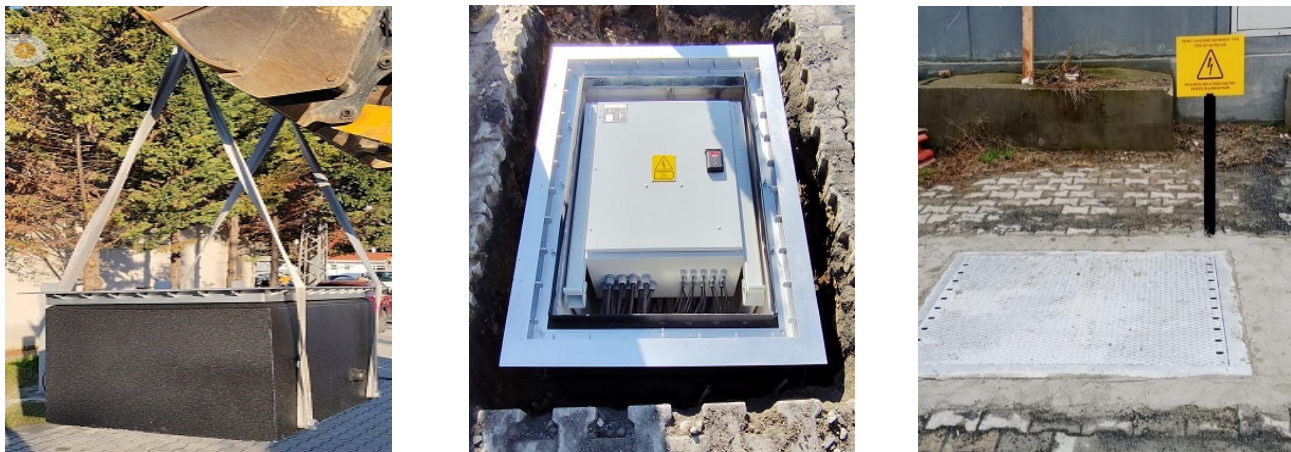
Figure 7. Underground LVDC Field Installation
