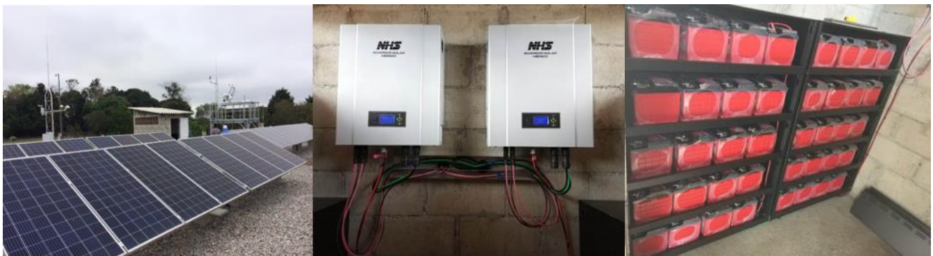
Fig 2: UTFPR PV-battery-grid-tie-system (PV-system-left/bidirectional inverters-center/battery bank-right) [14].
