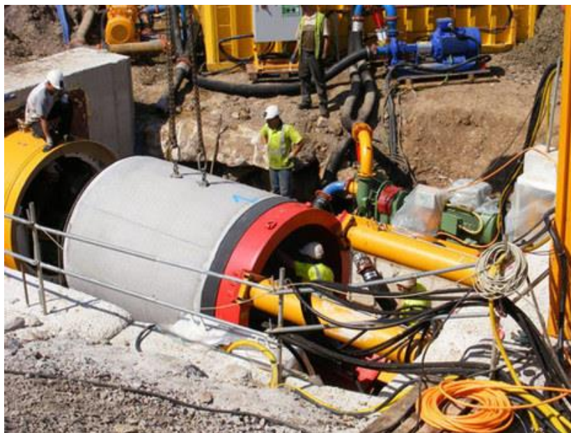
Fig. 1: Thrust Pit (Photo by Geosa)
