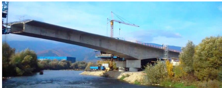
Fig. 1. View on the bridge No. 205 - final construction stage for the left cantilever – V1
