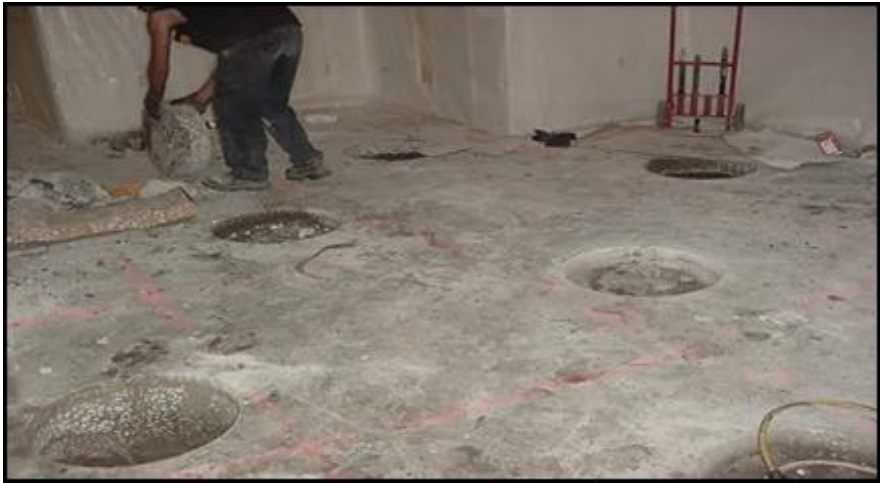
Fig. 2. Photograph of slab cores for the installation of conventional underpins
