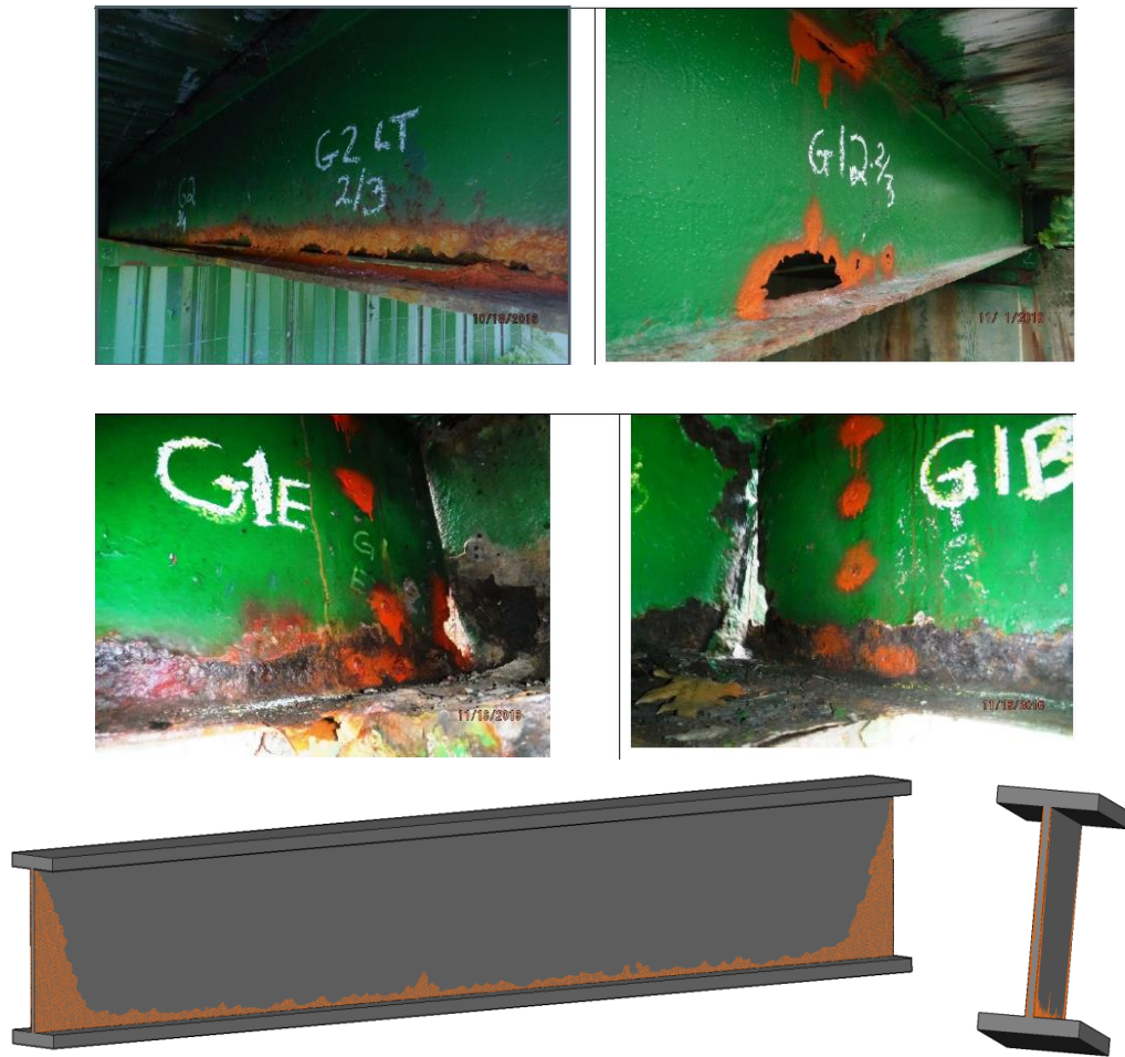
Fig. 1: Typical Steel Girder Corrosion at Web and Flange.
