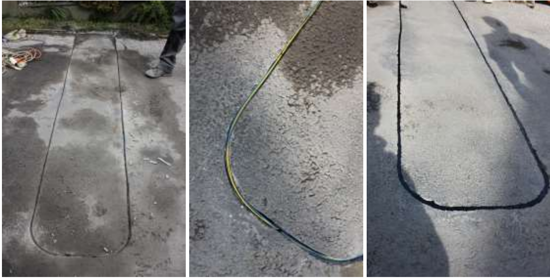
Fig. 2: a) Loop-shaped groove for measurement arms placement. b) Sensing optical fibers placed in the groove. c) Cold-casted groove with embedded optical fibers.
