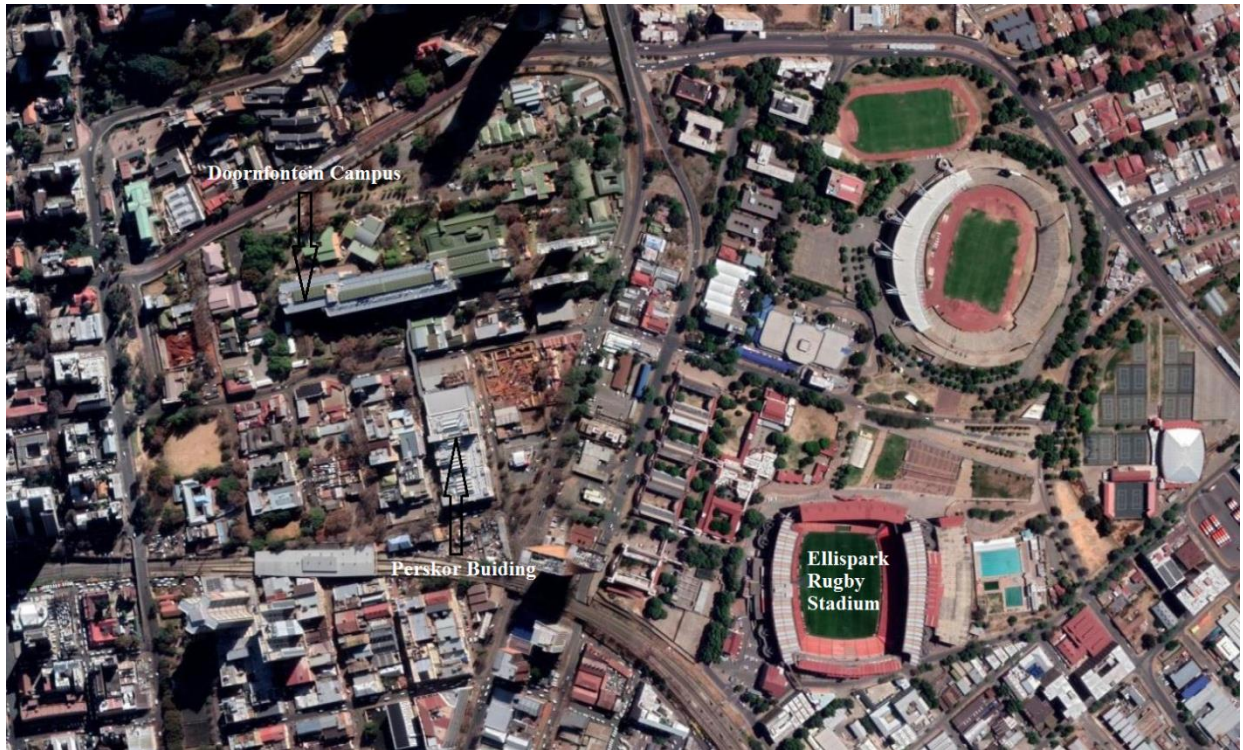
Fig. 1:Image found on Google Earth (23/12/20), showing the Doornfontein Campus and the Q/K building
