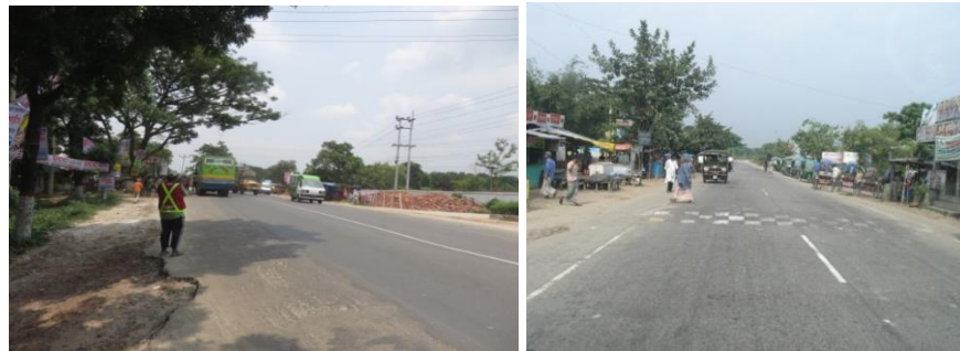
Fig. 1: A highway in Bangladesh with eroded edges (left) and faded markings (right), similar to 3 visited intersections.
