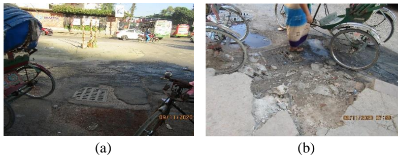
Fig. 2: An Urban Road in Dhaka City with Potholes (a) and edge Cracking (b).
