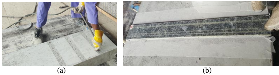
Figure 5: (a) Preparing the surface for EB application by sandblasting and cleaning; (b) Installing the EB-FRP.
