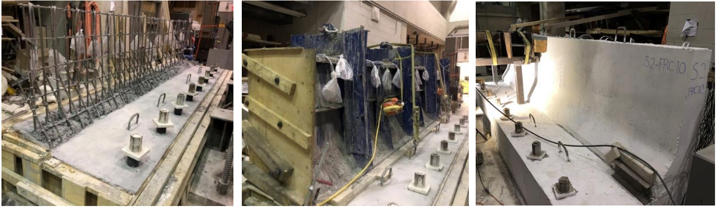
a) Wall reinforcement
