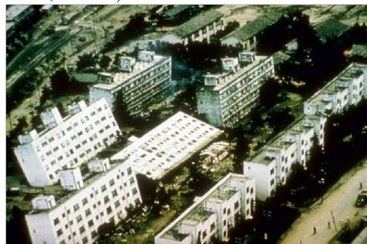
Fig. 1: Liquefaction in Niigata, Japan (1964)
