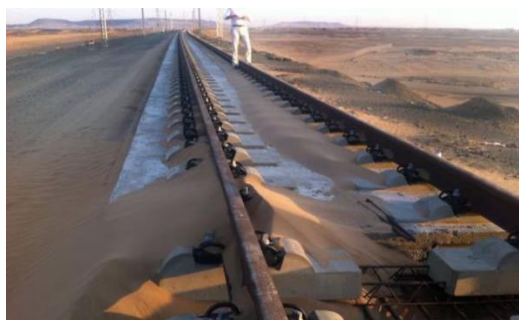
Fig. 4: Track under construction from Medina to Mecca [18].
