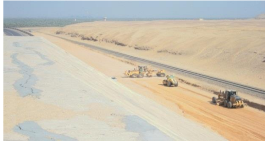
Fig. 2: Sand immigration particles to the existed track cause of construction works beside it.
