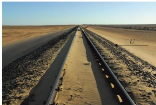
Fig. 1: Sand sedimentation induced by track line as an obstacle for wind direction [20].
