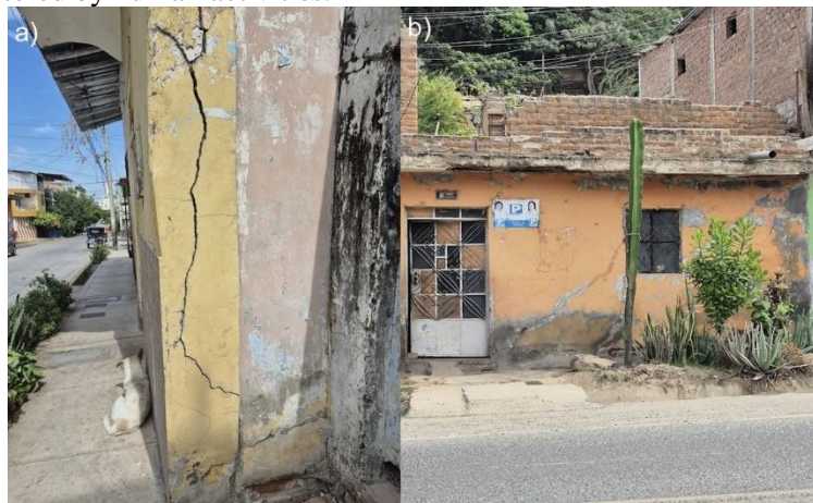
Fig. 1: Structures damaged by expansive clays in Sullana, Piura.
