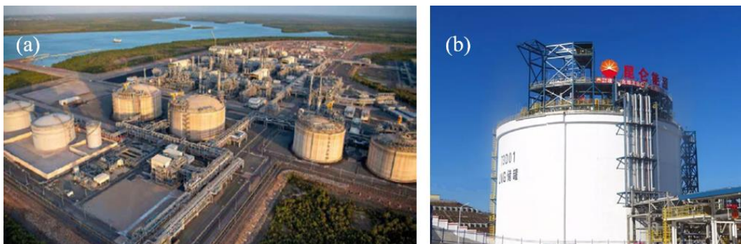
Fig. 1(a): LNG terminal facility [2], and (b). Typical full-containment LNG storage tank [2]
