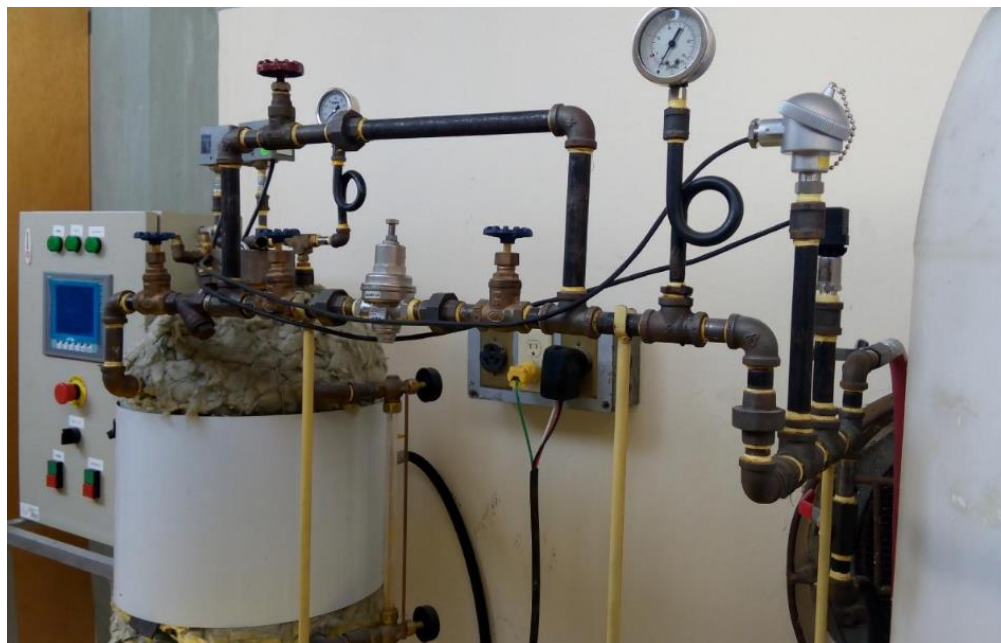
Fig. 2: Photograph the construction progress of the prototype SOEC.
