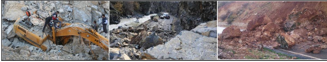
Fig. 1: Several rock failures that caused damage.
