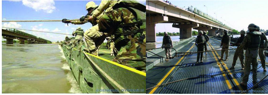
Fig. 1: An example of ribbon bridge installation process operated by human power [1].
